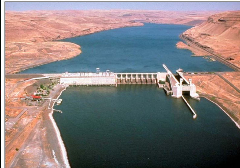
Tows on Columbia/Snake system in Pacific Northwest use unique locks with lifts over 100 feet. Tows can draft 14 feet.
