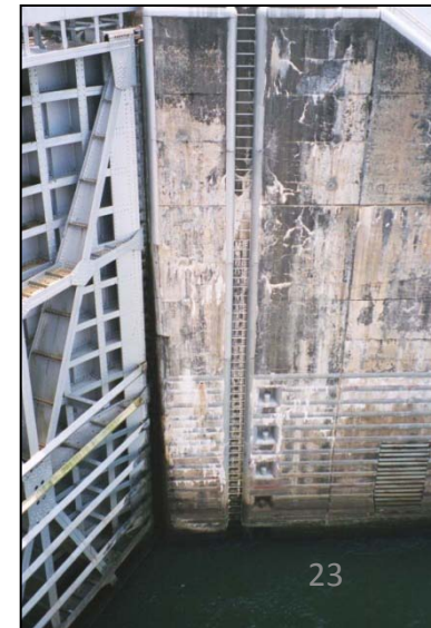
Lock wall deterioration, Chickamauga
