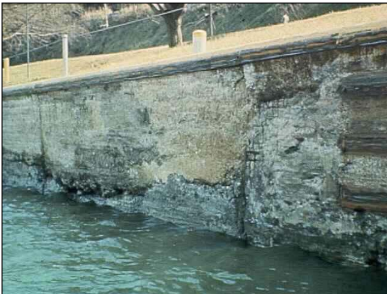
Crumbling lock wall, Lower Mon 3, opened in 1907
